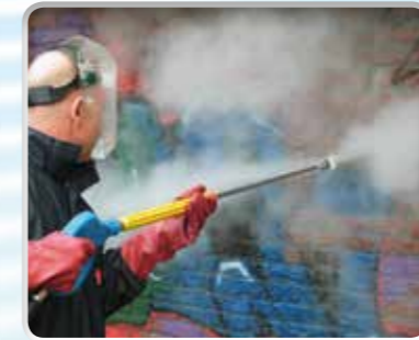
Graffiti removal: without chemicals
