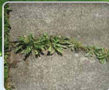
Weeds on pavement
